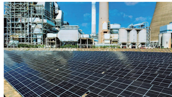
Zhejiang Company's photovoltaic project in Ninghai Power Plant
