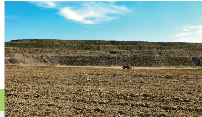
Work site of waste dump reclamation
