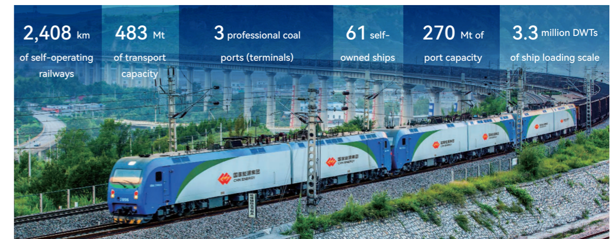
The 3+0 unit 10,000-ton train is driving on the Yelugou Bridge of the Shenmu-Shuozhou Line
