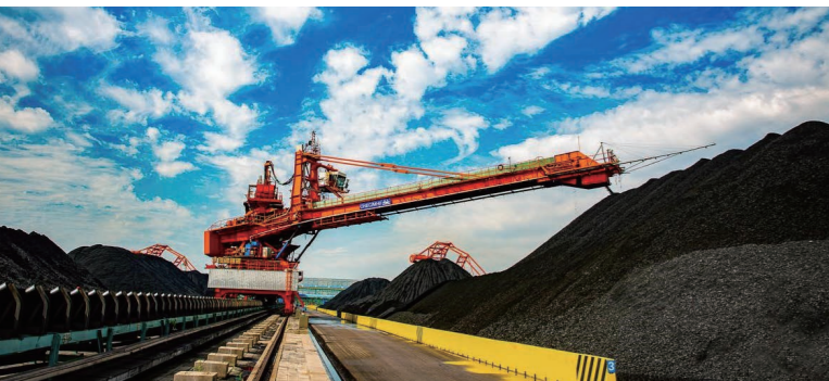
Unmanned coal stockpiling
