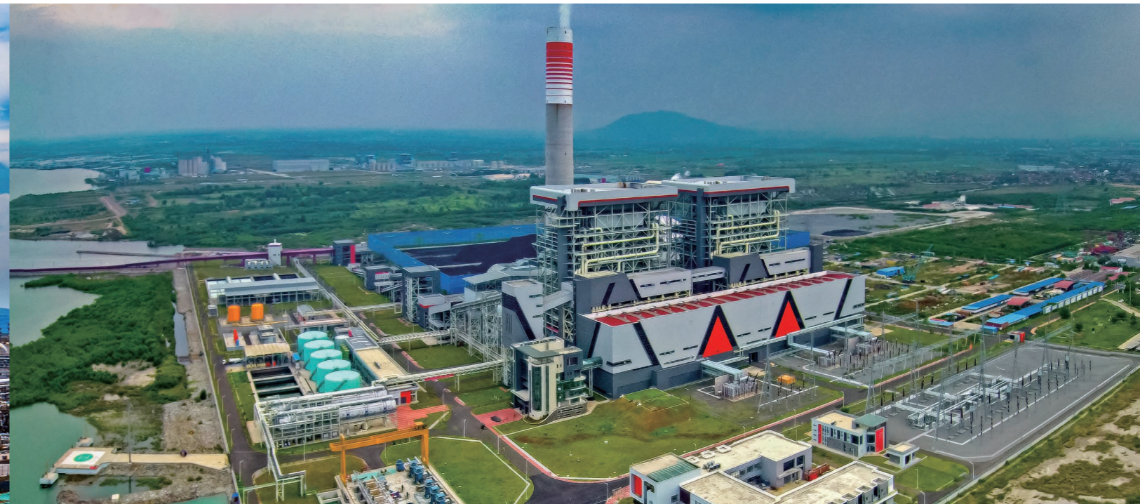
Guoneng Indonesia Jawa Power Generation Company was listed in the national key projects of Indonesia
