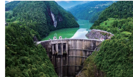
Luopoba Hydropower Station
