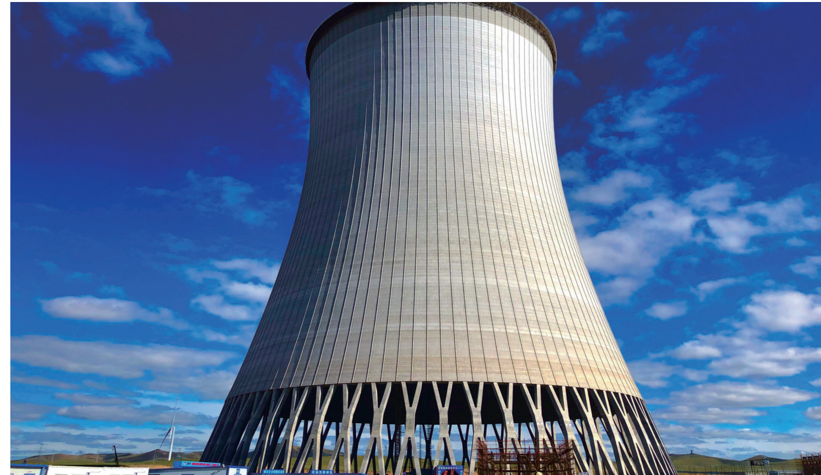
Guoneng Shengli Power Plant made a breakthrough in the cooling tower technology of “cooling water in place of chimney combining tower + integration of indirect dry cooling tower, chimney, first and second absorption towers, and wet electricity”, and the emission standards reached the “112” ultra-super-low emission target
