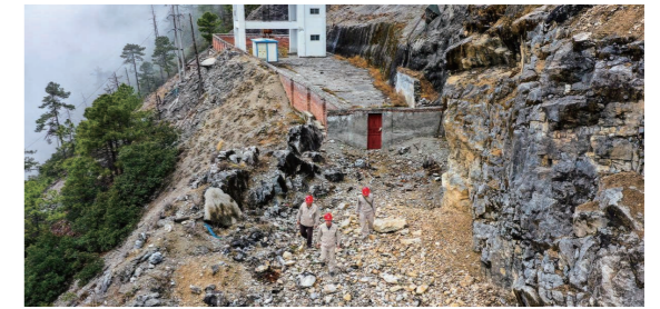
Safety patrol operation after the earthquake
