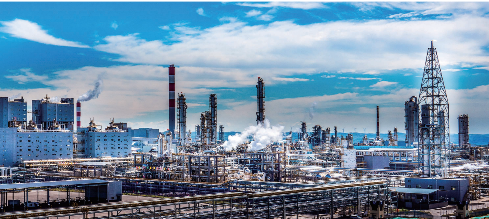
Yulin Chemical Company's 0.4 Mt/year ethylene glycol project was successfully put into production
